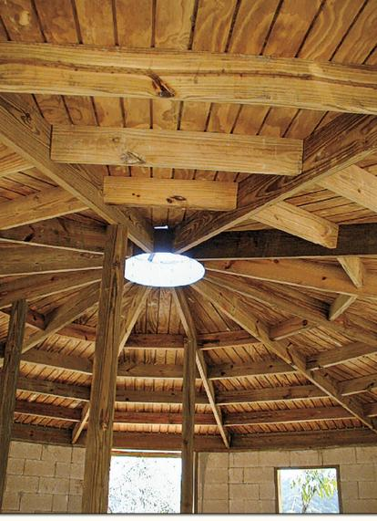
"A clear Plexiglas dome is located in the center of the roof over the steel ring..."
